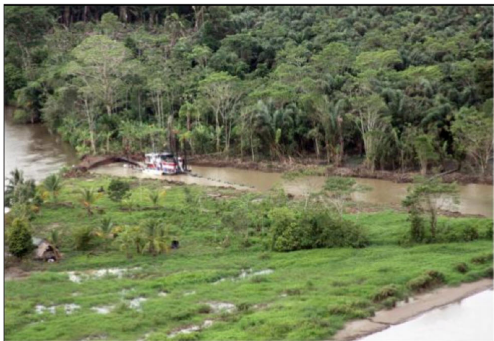
(e) 29 January 2011: dredger close to completing cut-off channel
