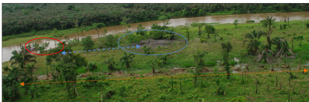
Figure Notes: This photograph shows the dredger (red circle), the depression left by the spoil pipeline linking the dredger to the spoil dump (blue line), and the area of floodplain wetland buried by dredge spoil (blue circle). The corridor cleared in preparation for digging of the 'Caño' is also visible (brown line).
