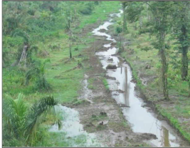
Figure I.35. Berms created by dumping of soil dug out to create the 'Caño'. Photograph taken on 5 April 2011.
