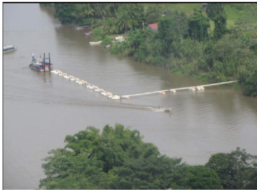
(a) dredge and spoil pipes at the Delta
