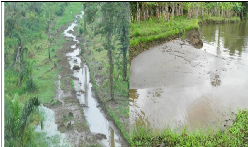
Figure 17. Erosion of the banks of the artificial canal and deposit of sediments in the confluence with the San Juan river. (Photo: A. Monge, April 2011).
