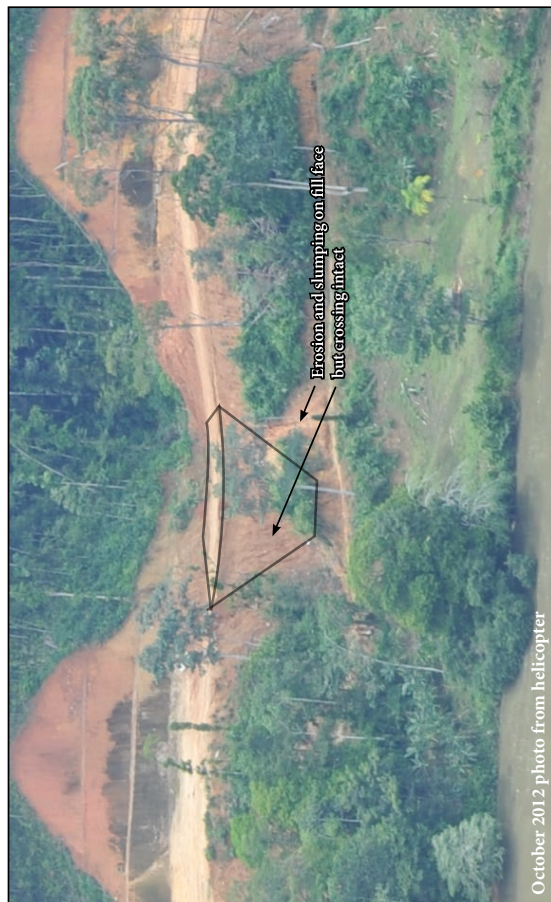
Gully on fill face (A) and erosion on backside of fill prism (B) (from Mende & Astorga 2013, p43).
