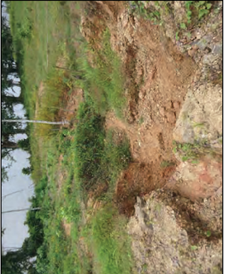
Photo 2.3. Failure and gulying of road fill prism with direct delivery to river (from Annex 5, Mende et al. 2013).
