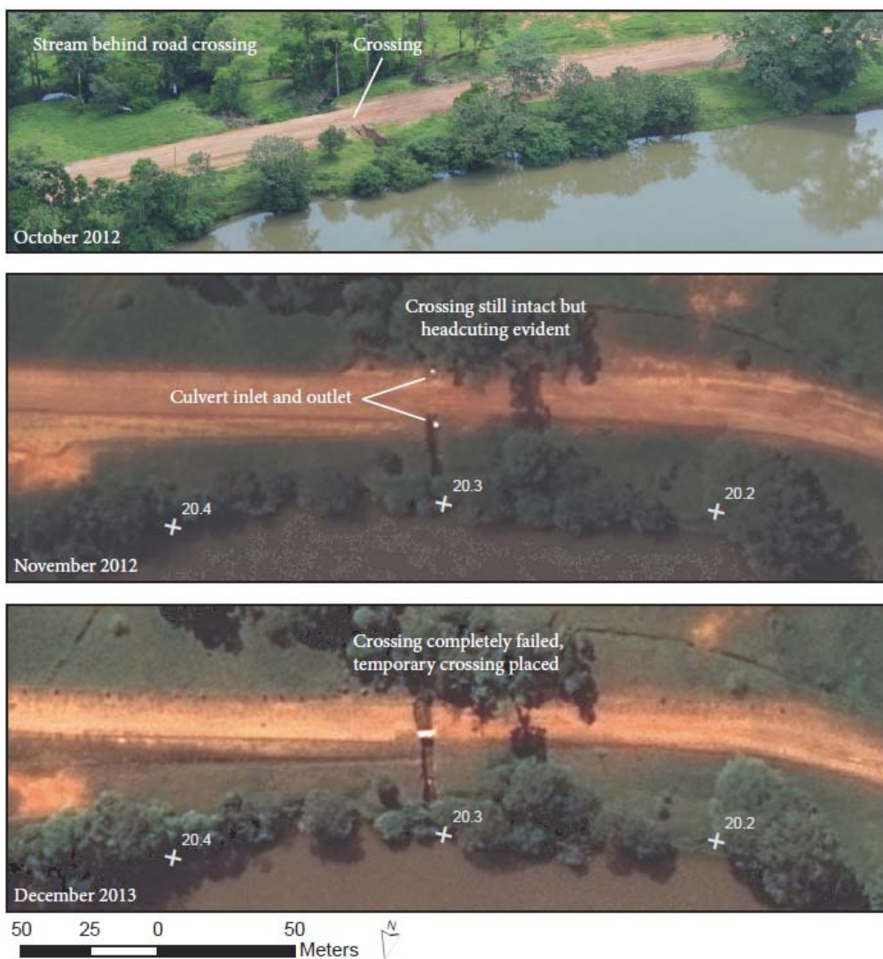
Figure 24. Helicopter and satellite imagery of failed fill crossing 20.3 km downstream of Mojon 2 border marker. a) The oblique helicopter photo of October 2012 shows evidence of headcutting. b) The November satellite 2012 imagery shows the same situation: headcutting but the fill still mostly intact. c) By December 2013, satellite imagery shows the crossing had failed completely. A temporary single-track crossing had been placed over the channel, and fill material had been placed in the channel to re-narrow the crossing, but the culvert had not been replaced and water was flowing freely over the loosely compacted material. The plastic pipe culvert washed out and was transported down to the Río San Juan along with the eroded sediment, as illustrated in Figure 25.
