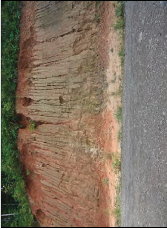
Photo 3. Rills on cut slope (from Mende & Astorga 2013, p36)
