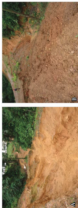
Gully on fill face (A) and erosion on backside of fill prism (B) (from Mende & Astorga 2013, p43).
