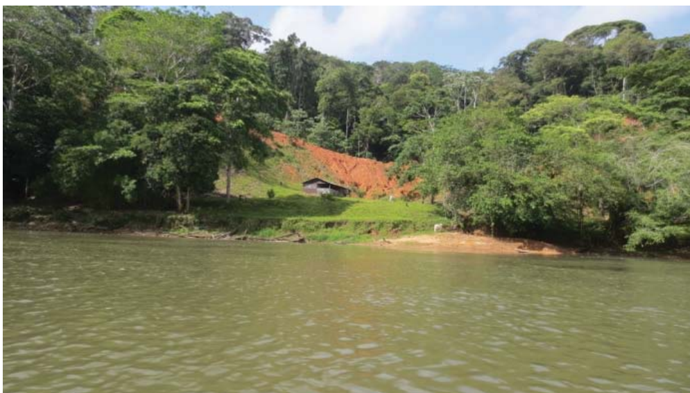
PHOTO 2 - Location: RKM 18.2 to 18.3 (from boat, May 2014). Formation of sediment delta from failed earthen fill stream crossing and other erosion.
