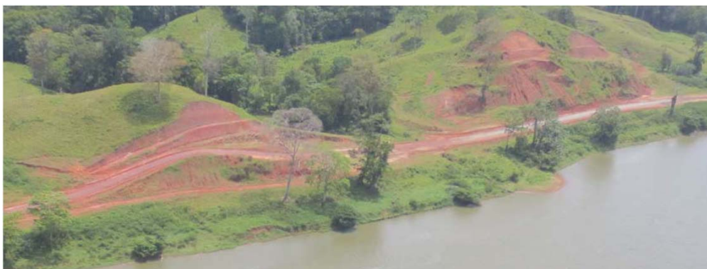
PHOTO 5 - Location: RKM 21.4 to 22.1 (from helicopter, May 2014). Section of the roadway that is too close to the river. The steep cuts that have been made to construct the road and lack of erosion and sediment controls have resulted in sedimentation of the river. The terraces constructed in the slope provide little control of erosive effects of water from storm events as evident from the erosion gulches of the face of the cuts into the hills.
