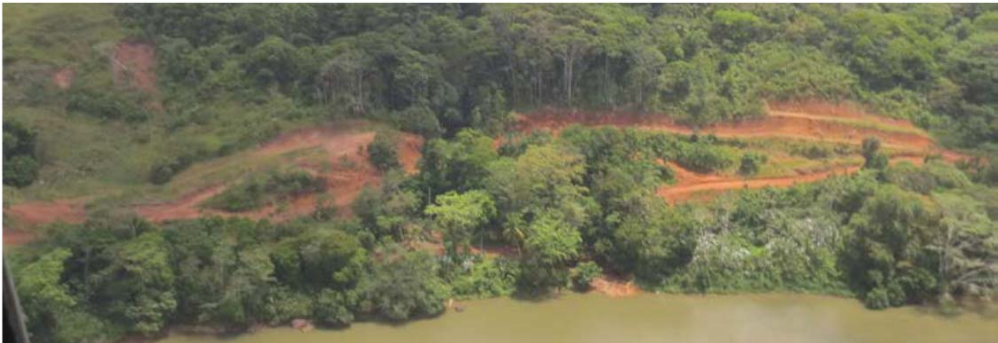
PHOTO 11 - Location: RKM 23.6 to 24.5 (from helicopter, May 2014). Areas of excessive tree cutting used to construct two routes in this area.
