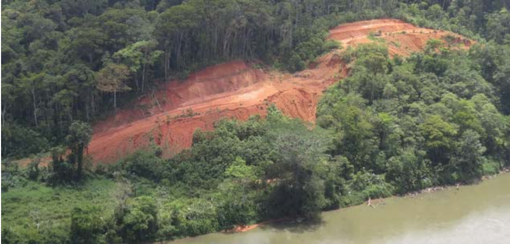
PHOTO 10 - Location: RKM 16.1 to 16.5 (from helicopter, May 2014). Excessive removal of trees to construct the roadway that has resulted in exposed and unprotected slopes leading to slope instability.
