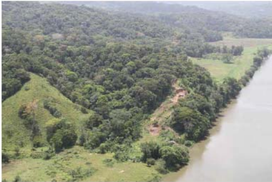
Figure 8. May 2014 oblique aerial view of the failing slope 1 km downstream of El Jardin (Rkm 36.4)
