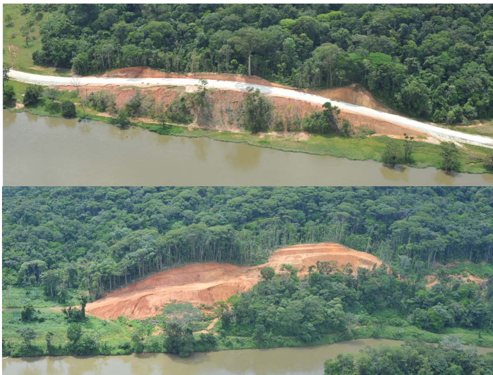
Figure 22. Examples of sidecasting fill material. a) Severely Eroding Site 4 (Rkm 8.2-8.7) (photo from helicopter over north bank of Rio San Juan, October 2012). b) Severely Eroding Site 8 (Rkm 16.1-16.4) (photo from helicopter over north bank of Rio San Juan, October 2012). It is clear from the loose, failing nature of the fill slopes that the bulldozers simply dumped the material down the slope below, creating an unstable slope of loose fill vulnerable to landsliding, gullying, and rilling.
