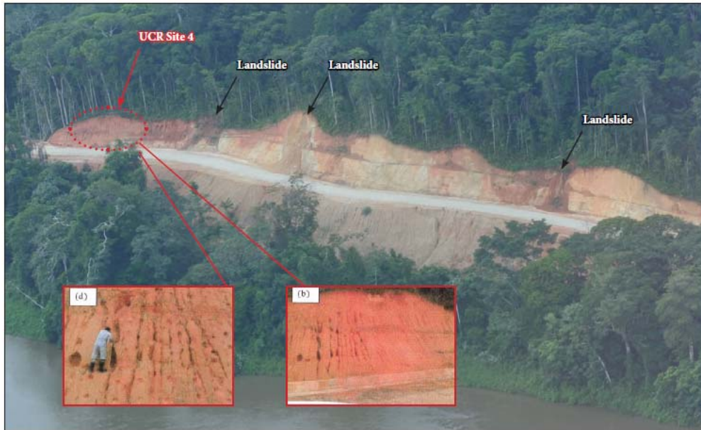
Figure 28. Context of UCR's Site 4 within a larger complex of eroding features from Rkm 10.4 to 11.3. a) Oblique aerial photograph from helicopter, October 2012, showing multiple landslides to the right (west) of the site selected for detailed study by UCR. b) Detail of the same photograph, showing larger eroding features in cutslope, similar to the rills measured by UCR but larger, as well as two nearby landslides. The UCR Report (Annex 1) presented only photos showing close-up views of the section of the rilling cutslope where UCR made its measurements (inset). Note that the UCR photo labeled "b" ended just to the right of much larger eroding features in the cutbank, similar to but larger than those measured by UCR.
