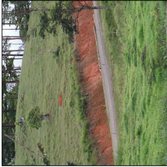
Photo 3. Eroding outslope adjacent to blocked drainage (view from riverboat, October 2013).
