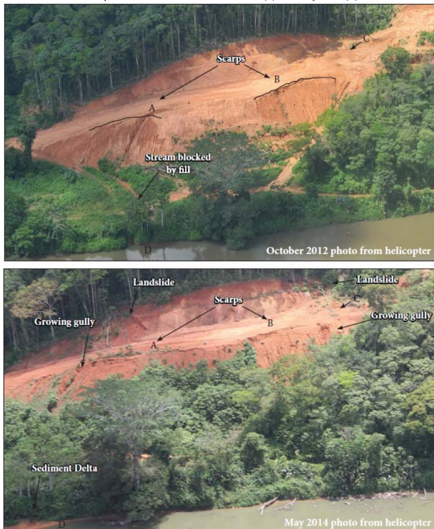
Figure 19. Eroding Site 8.2, 16.2 km downstream of Mojon II. Oblique aerial views from October 2012 (a) and May 2014 (b).
