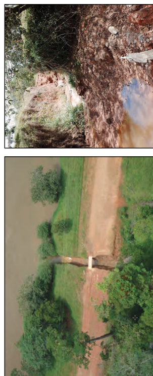
Photo 2. Failed road crossing at RKM 21.3 (from Mende & Astorga 2013, p.53). Report notes plans to install a larger diameter culvert.
