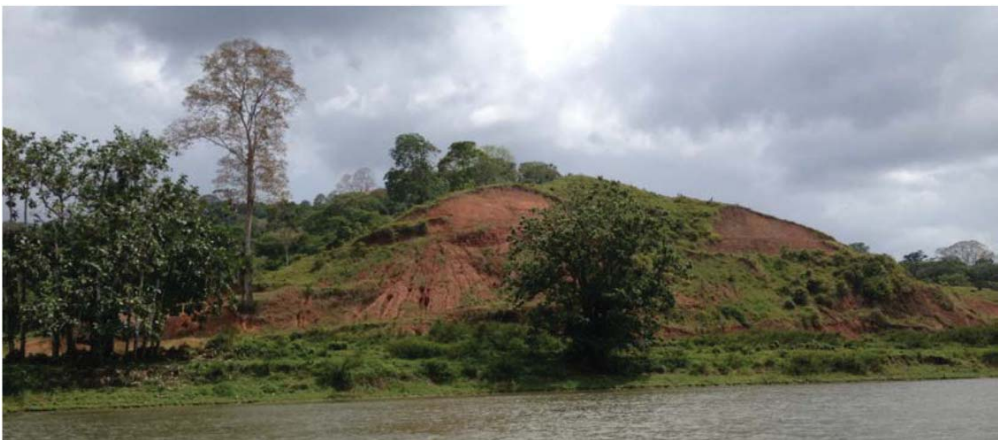
PHOTO 7 - Location: RKM 7.4 to 7.9 (from boat, May 2014). An example of lack of proper design and planning process that has located this section of the roadway through undesirable topography. This includes areas that are too steep, too uneven, or too high in comparison to the surrounding environment. The topography in combination with the type of erodible soils combined to create unstable slopes and erodible conditions that have resulted in the sediment loading to the river.
