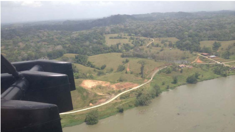
PHOTO 6 - Location: RKM 7.4 to 7.9 (from helicopter, May 2014). An example of lack of proper design and planning process that has located this section of the roadway through undesirable topography. This includes areas that are too steep, too uneven, or too high in comparison to the surrounding environment. The topography in combination with the type of erodible soils combined to create unstable slopes and erodible conditions that have resulted in the sediment loading to the river.
