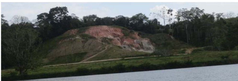
PHOTO 12 - Location: RKM 7.4 to 7.9 (from boat, May 2014). Borrow pit used for extracting soils for the construction of the roadway. The pit constructed in high topography has been left open and subject to erosion from precipitation events without appropriate BMP.
