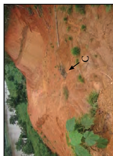
Steep and unsta- bles cut and fill slopes (from Mende & Astorga 2013, p40).
