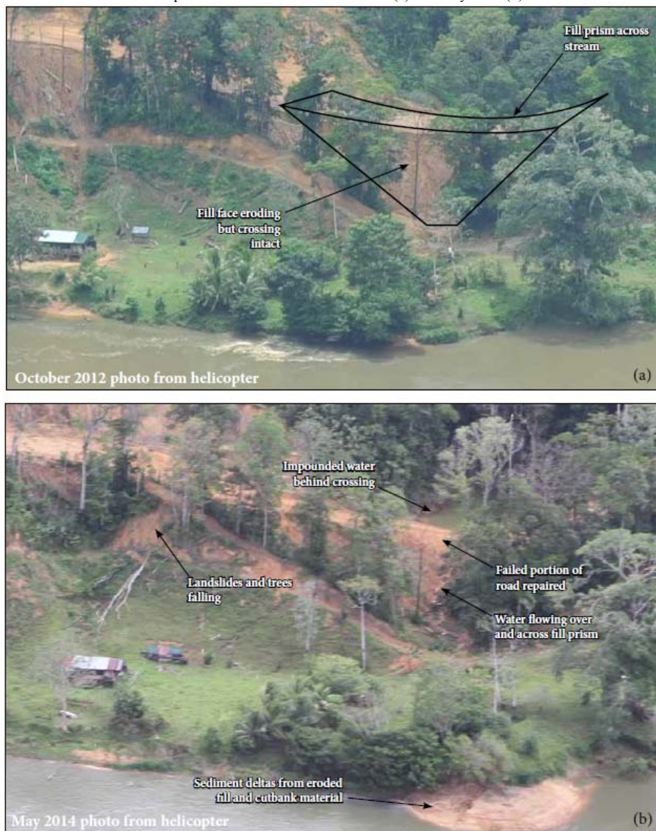
Figure 10. Eroding Site 9.4, 18 km downstream of Mojon II. Oblique aerial views from October 2012 (a) and May 2014 (b).
