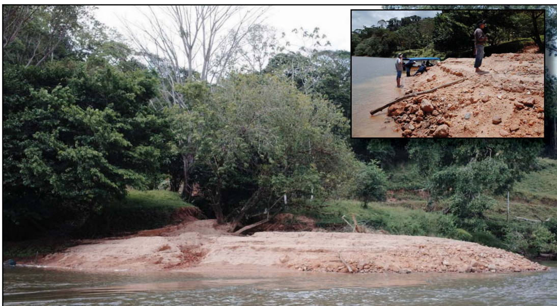
Delta deposit below Erosion Site 9.4. Ecological Sampling Site 2a.
