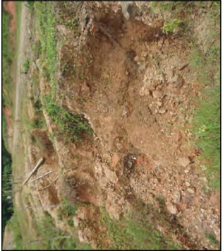
Photo 2.3. Failure and gulying of road fill prism with direct delivery to river (from Annex 5, Mende et al. 2013).
