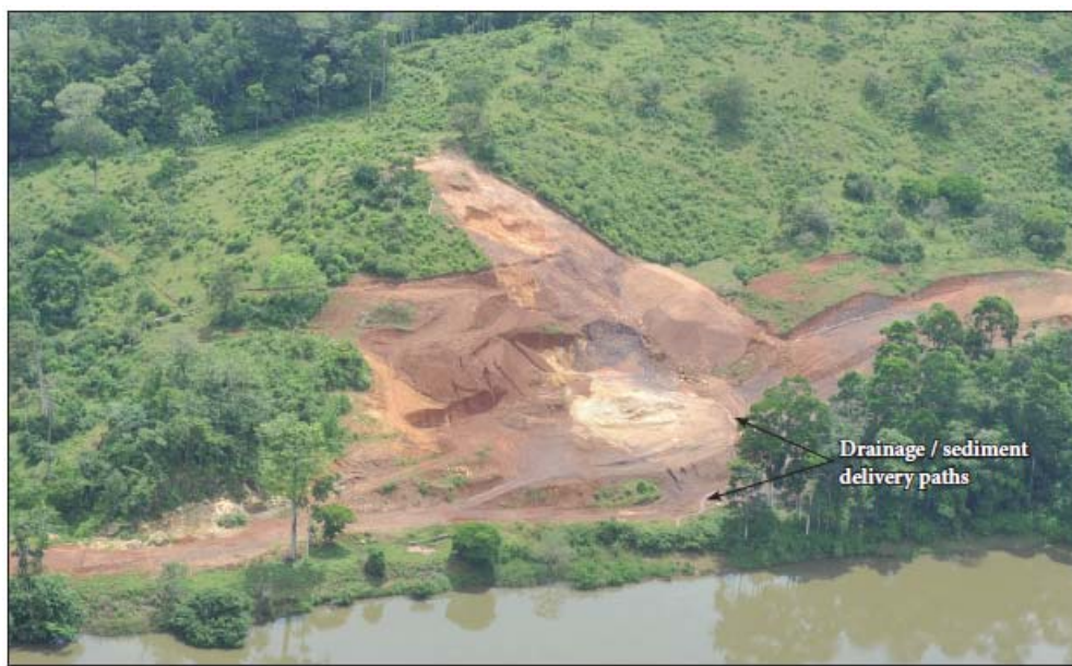
Figure 23. Surface erosion of a quarry for road construction materials located at Rkm 25.3 km (downstream of Mojon II). No erosion control, slope stabilization, or drainage measures were visible as of May 2014. Sediment-laden runoff from the exposed quarry surfaces drained towards the Río San Juan, and by May 2014 had eroded a small channel to carry this runoff and sediment into the Río San Juan. (Photographs taken from helicopter over the north bank of the Río San Juan.)
