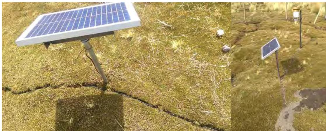
*Figure 4-3. Solar panel, tipping bucket and buried cables of the Quebrada Negra Wetland meteorological station.*
