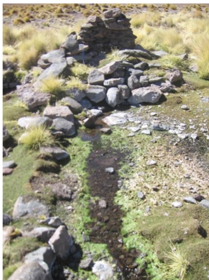
a) Dam and spring protected with rock
