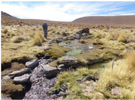
a) Union of collector canals of springs 01 to 07.
