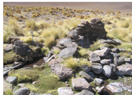
b) Catchment work with protection to collect water from the spring.
