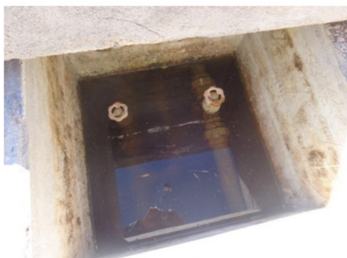
a) Interior of the masonry chamber with pipes and gate valves.
