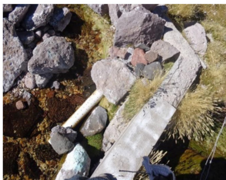
a) Pipe to divert water to the pond.
