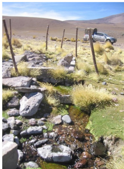
b) Springs protected by a dam of old rocks and recent masonry.
