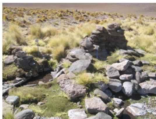
b) Catchment work with protection to collect water from the spring.
