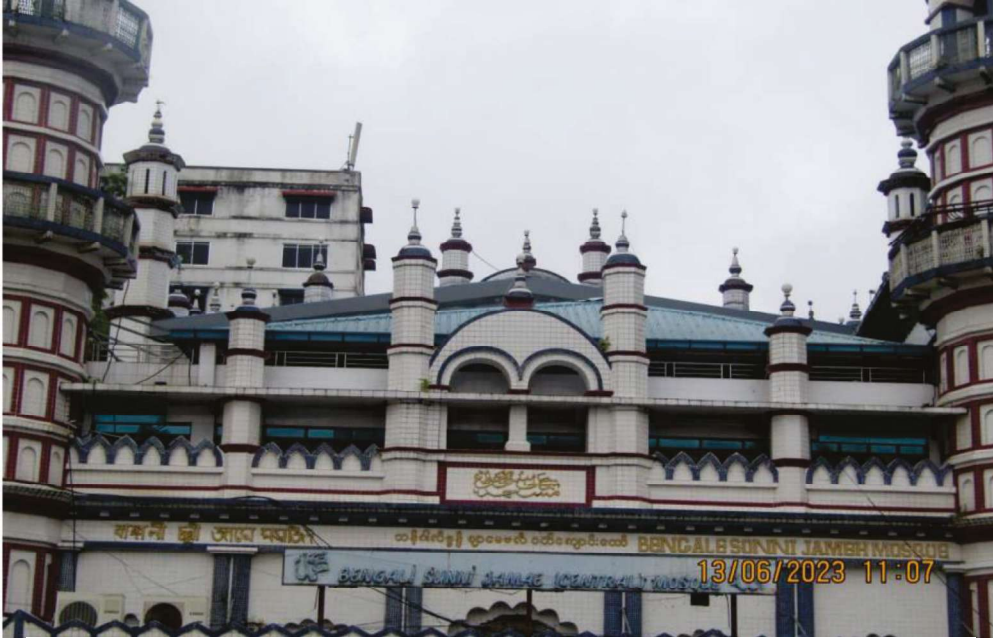
Front view (Close up) of the Main Signage of the Mosque
