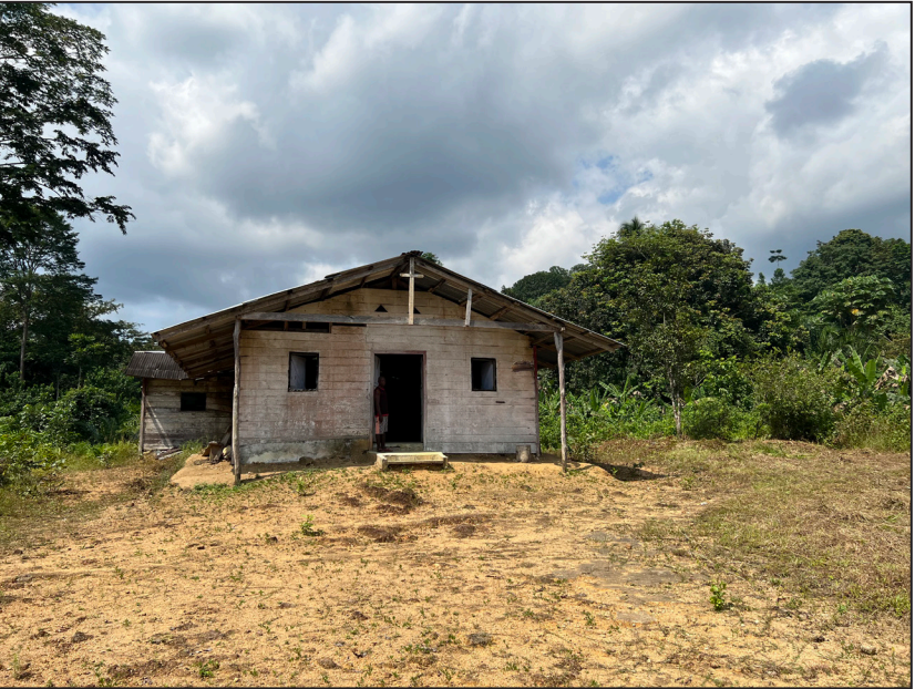
Annex P.U17 Church
