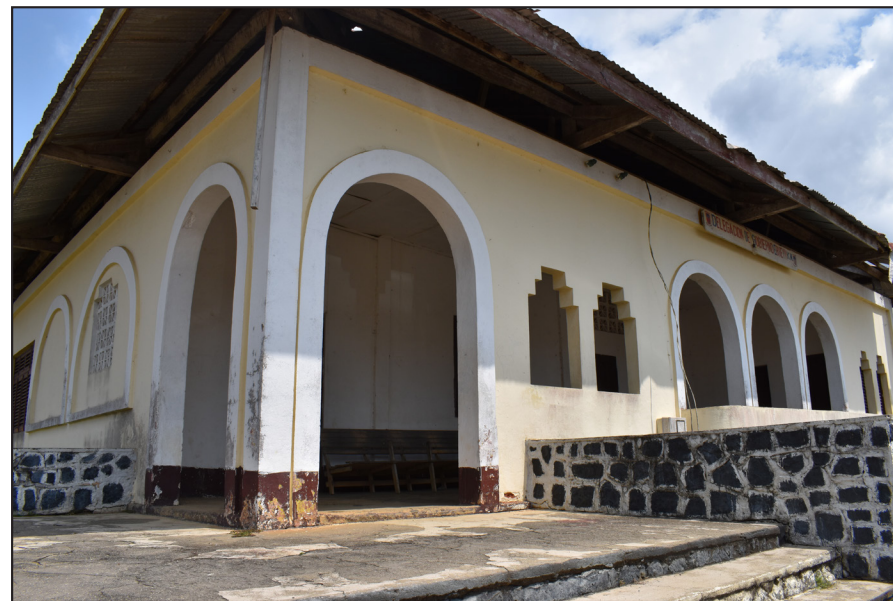
Annex PE16 Spanish Colonial Administrative Building (now Delegación de Gobierno de Ebebiyin K.N.)
