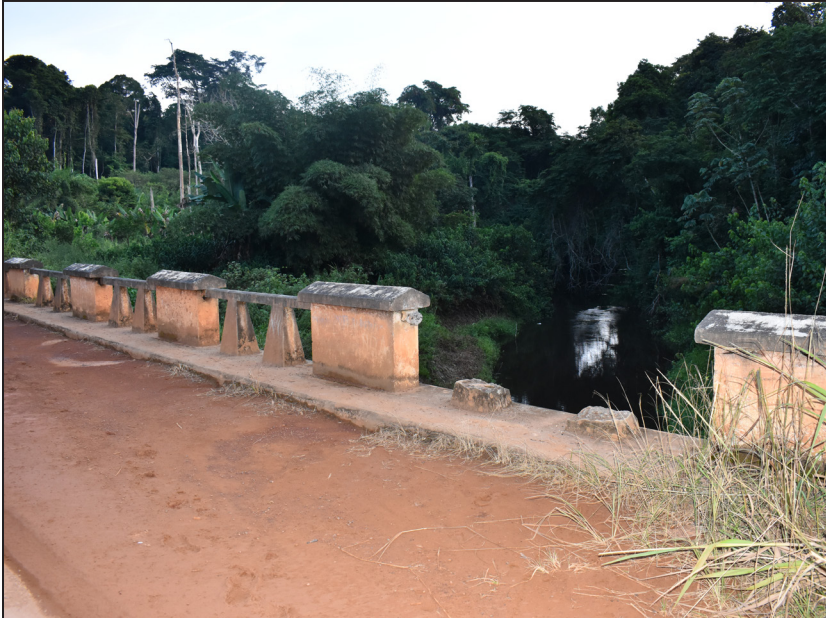
Annex P.K1 Bridge over Abos River
