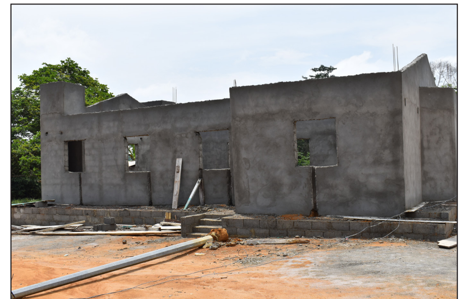
Annex P.K34 Church (Under Construction)
