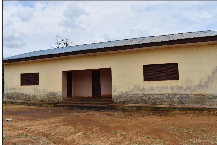
Annex P.K24 School
