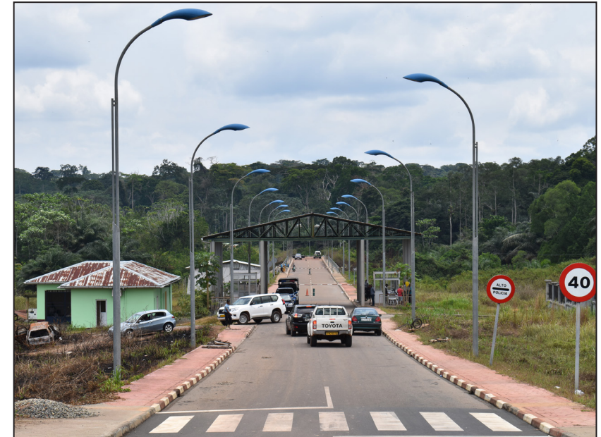
Annex P.E9 Ebebiyin Bridge Overview (2)
