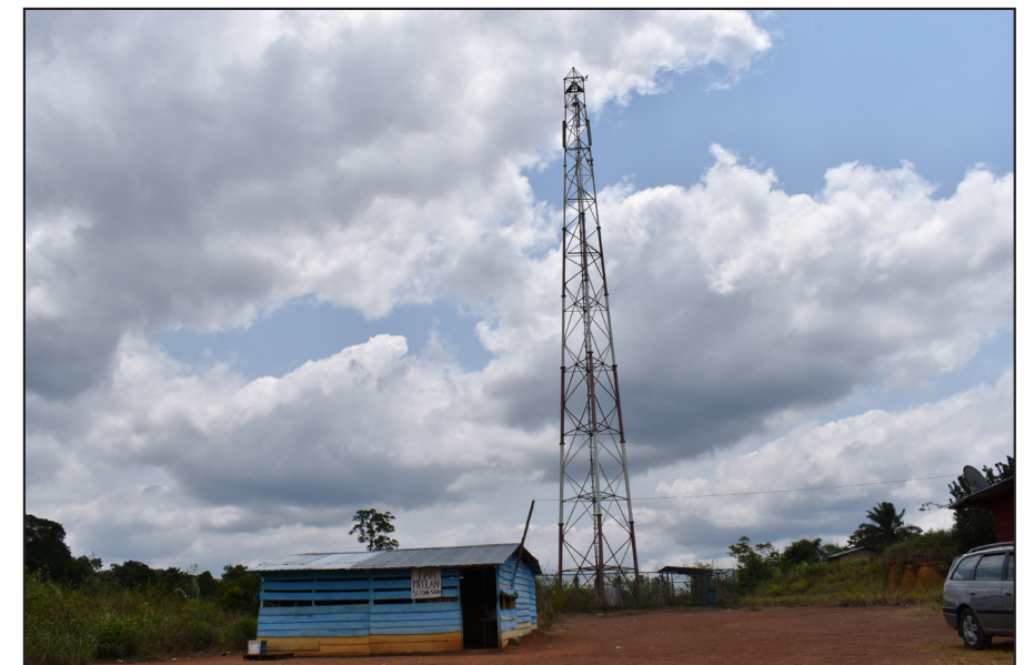
Annex P.E6 GETESA Tower (Equatorial Guinea Telecommunications LLC)
