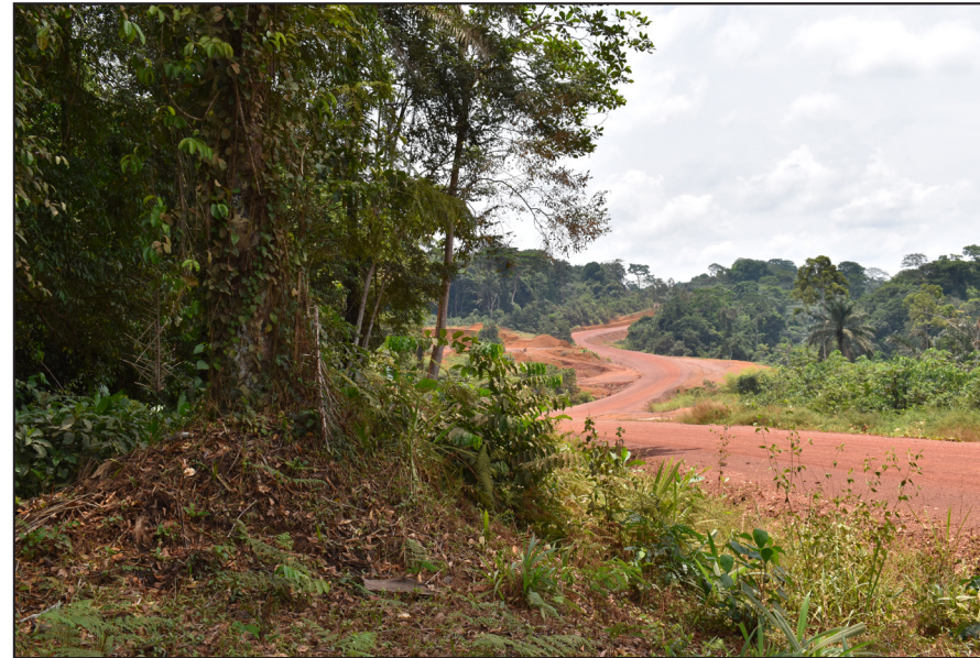
Annex P.K30 Road Improvement (1)
