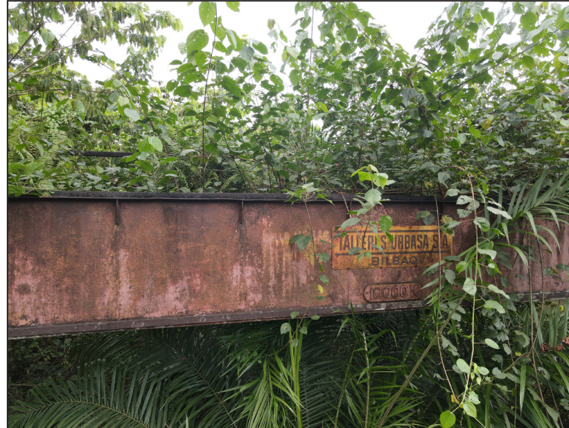
Annex PU11 Crane
