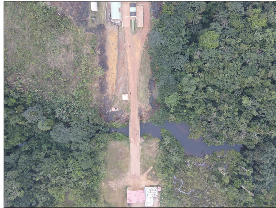
Annex P.MO8 Mongomo Bridge Overview (1)
