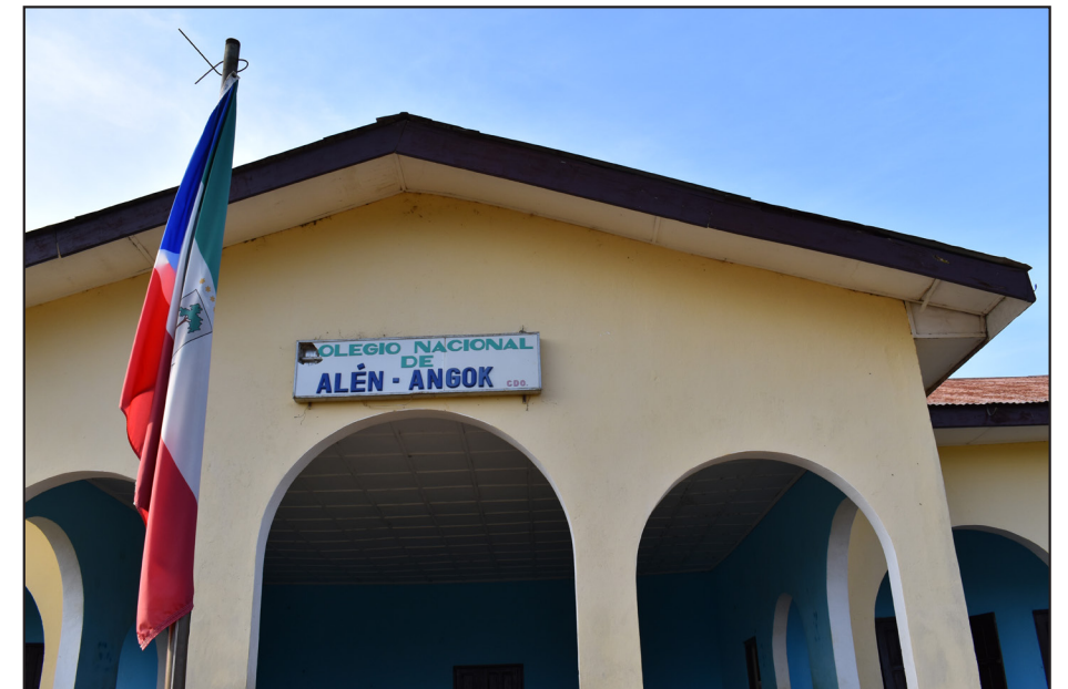
Annex P.K4 School
