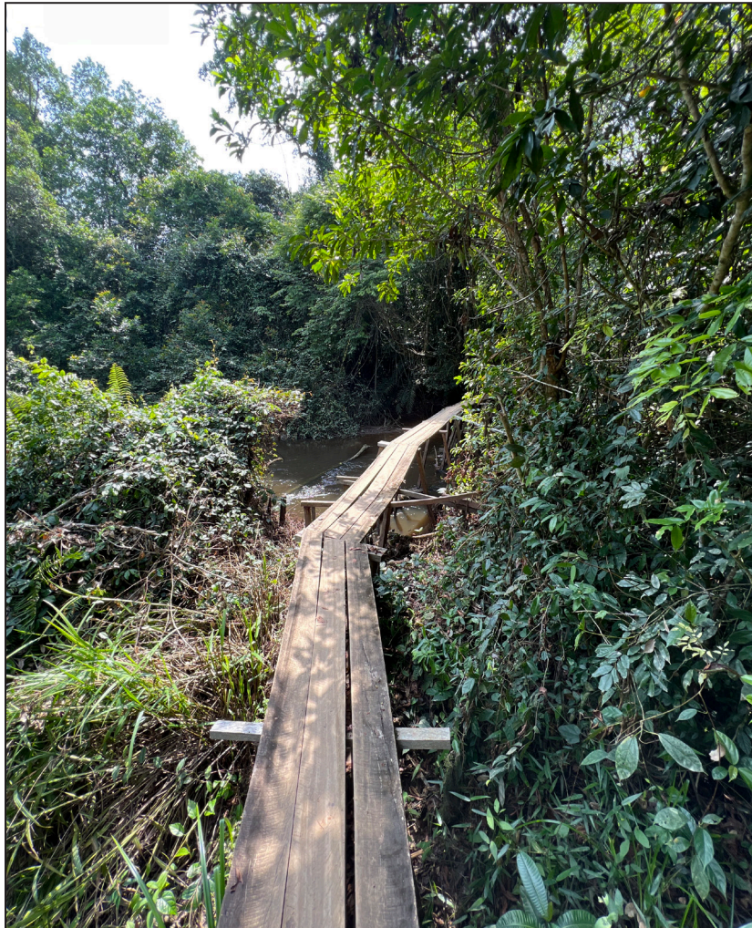
Annex P.K11 Footbridge
