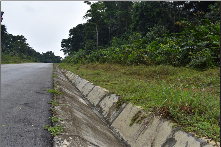
Annex P.K37 Paved Road / Guttering
