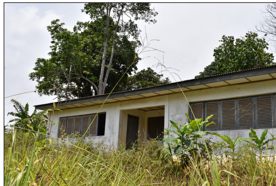
Annex P.K33 School
