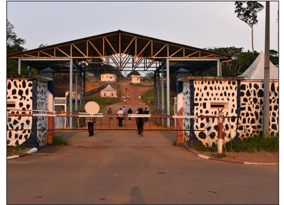
Annex P.MO9 Mongomo Bridge Overview (2)
