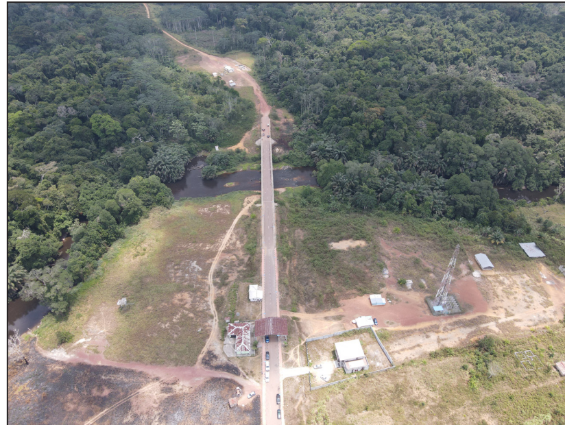
Annex P.E8 Ebebiyin Bridge Overview (1)
