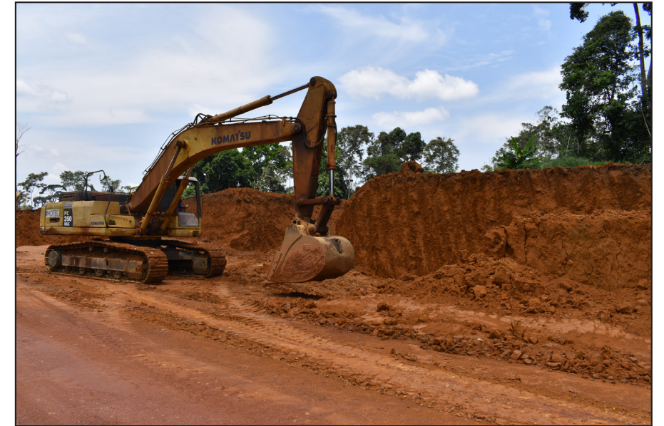
Annex P.K31 Road Improvement (2)
